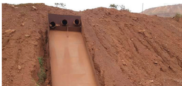
Fig. 5(a). GI sheets with drainage arrangements
