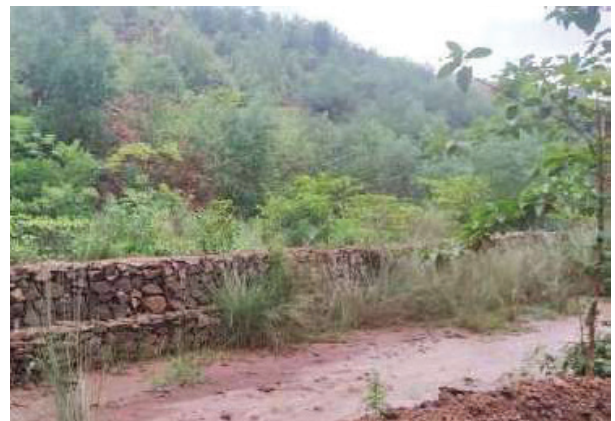
Fig. 3. Biologically reclaimed part of existing external OB dump along with retaining wall and garland drain
